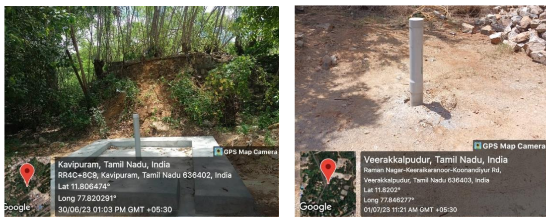
Figure 3.10. Geotagged photographs of the new borewells constructed in Plant 1 and Plant 3
